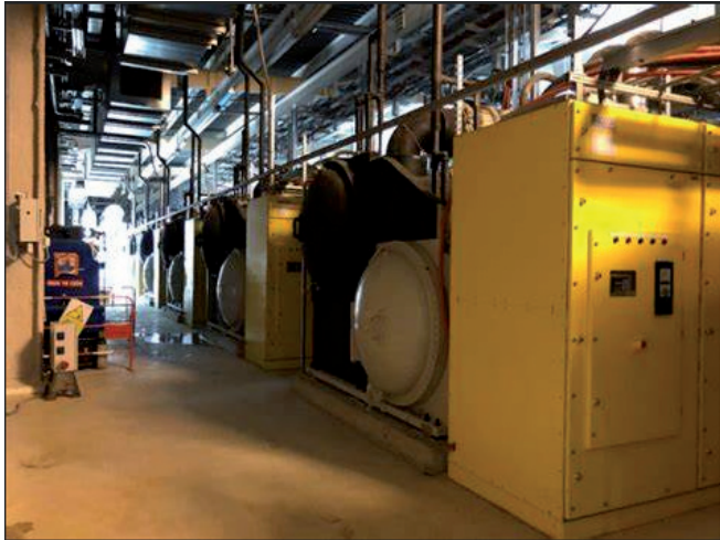
Figure B.1.5: Water cooled chillers.
